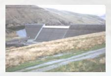
Willow Creek Dam, the world's first all roller compacted concrete structure
