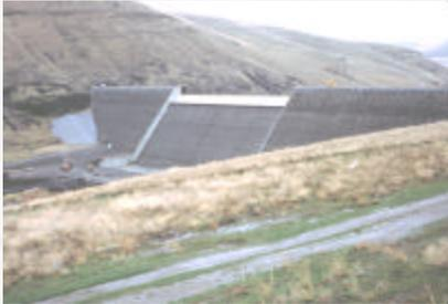
*Willow Creek Dam, the world's first all roller compacted concrete structure*
