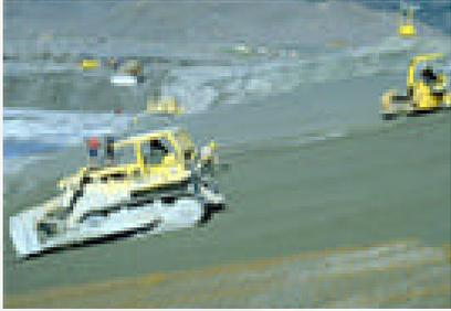
Mount St Helens Sediment Retention Structure, roller compacted concrete
